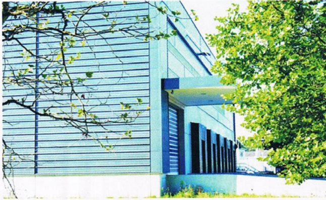
Quelle: Hoffmann Facility Management
