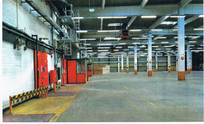
Quelle: Hoffmann Facility Management
